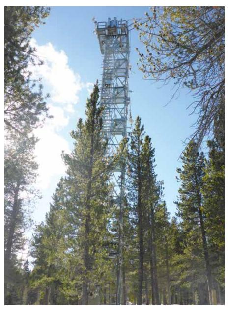
NEON's tower in Rocky Mountain National Park resembles the proposed tower that would be installed in Yellowstone National Park. The tower, used to monitor air temperature, humidity, precipitation, air quality, soil chemistry and other data, is proposed at 70 feet tall, with an alternative height of 59 feet. It would be powder coated green. PHOTO COURTESY OF NEON
