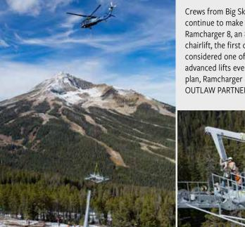
Crews from Big Sky Resort and Doppelmayr continue to make progress installing Ramcharger 8, an 8-person, high-speed, D-line chairlift, the first of its kind in the world and considered one of the most technologically advanced lifts ever built. If all goes according to plan, Ramcharger 8 will open on December 15. OUTLAW PARTNERS PHOTOS
