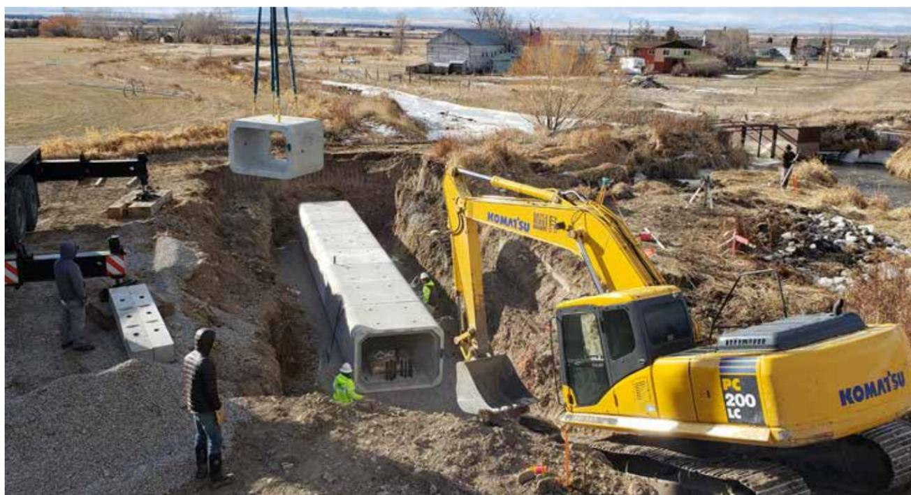
The second phase of the restoration project on Dry Creek involves a fish ladder that runs beneath an existing irrigation ditch. It will give migratory fish access to the cold, clean waters of the tributary in the summer months when warm temperatures can threaten coldwater fish. PHOTO COURTESY OF SCOTT GILLILAN
