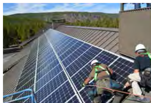
Solar panels are installed on one of Yellowstone National Park Lodge's buildings as a part of their sustainability program. PHOTO COURTESY OF YELLOWSTONE NATIONAL PARK LODGES
