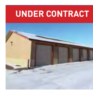
Car Park Condo Unit E7 Bozeman, MT 23'x11'x10' / $24K
