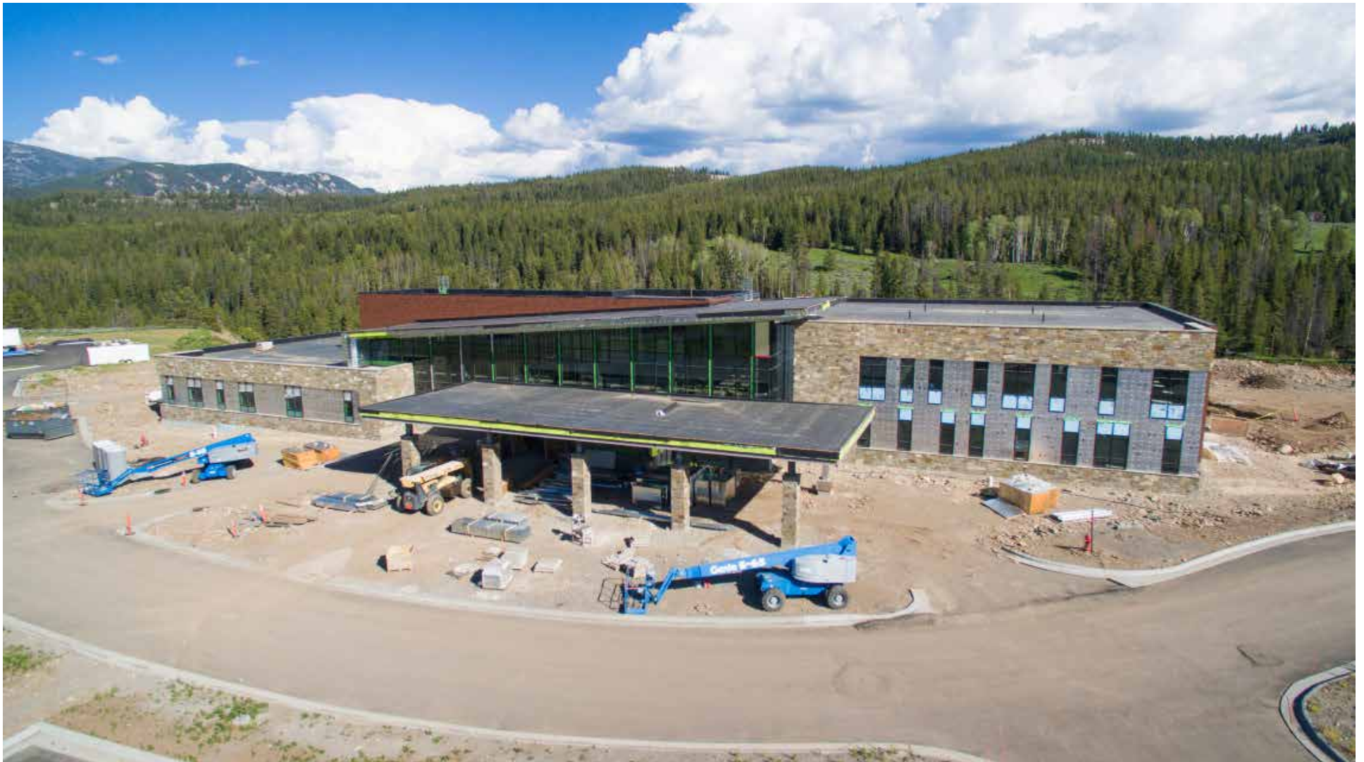
The Big Sky Medical Center under construction. The Bozeman-Health-run hospital opened its doors on Dec. 12, 2015.
