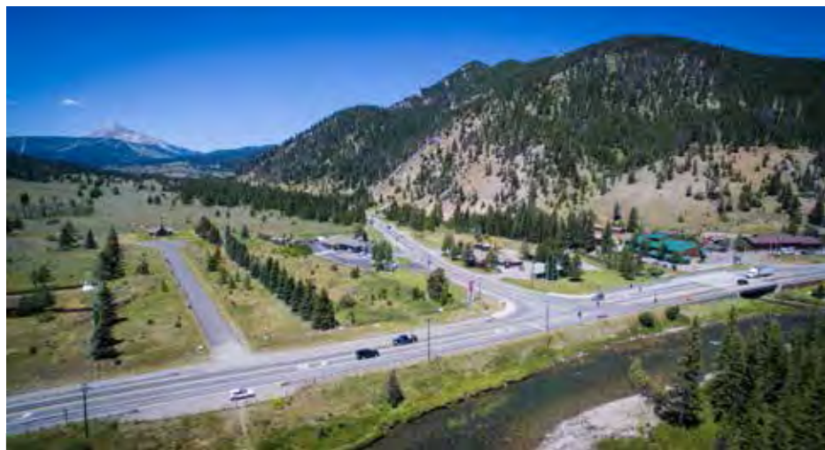
Funding from the federal TIGER grant and the settlement payment from developer A2LD will lead to upgrades along Lone Mountain Trail beginning next summer. Once turning lanes are completed at the intersection of Ace Hardware and the easternmost entrance of the development, construction can begin on the Powder Light subdivision. OUTLAW PARTNERS PHOTO
