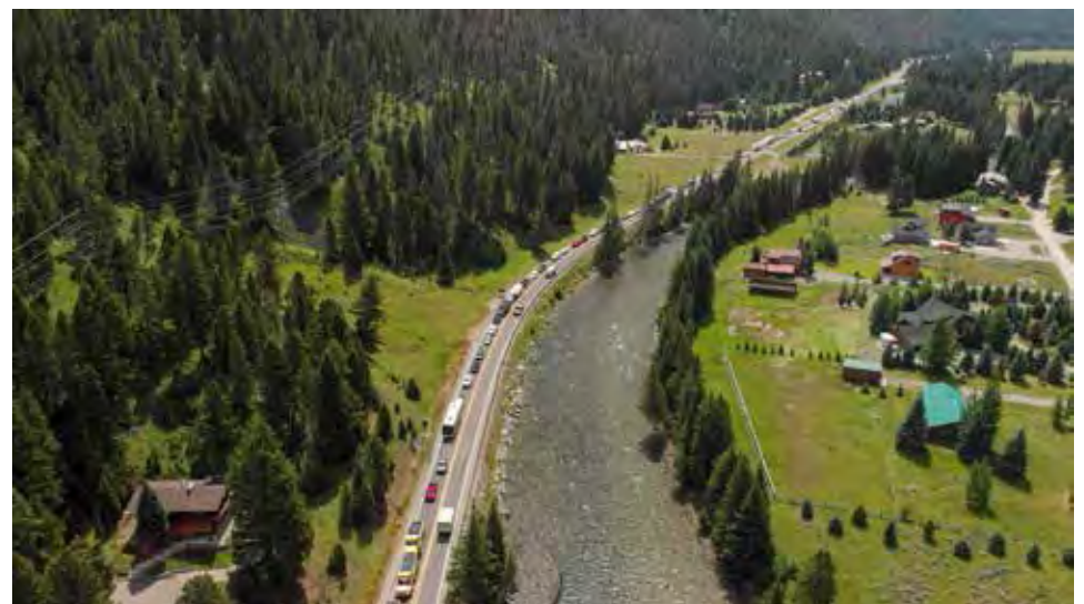
A long line of cars travel on Highway 191 between Big Sky and Bozeman. Canyon traffic is one tangible sign of the rapid growth occurring in the area. OUTLAW PARTNERS PHOTO
