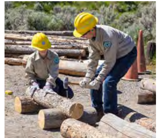
Participants of the 2018 Youth Conservation Corps build bumper logs at Boiling River parking lot. NPS PHOTO
