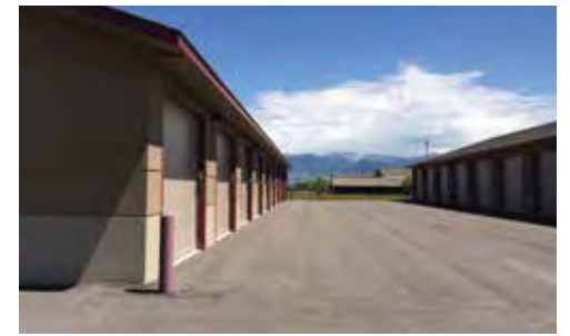
Airport Garages Bozeman, MT $29.9K per unit Taking reservations for building G
