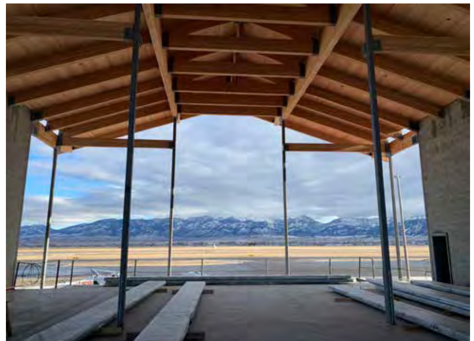
Bozeman Yellowstone International Airport’s new terminal building is well underway. A number of local artists have expressed a desire to donate or exhibit various works of art for its walls once it is finished. PHOTO COURTESY OF LISA BURGWIN
