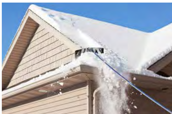
Large amounts of snow should be removed in order to prevent ice dams and reduce excess weight. PHOTO COURTESY OF FIRST SECURITY BANK
