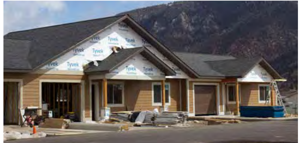
Volunteers from Habitat for Humanity International, AmeriCorps, Suffolk Construction and Lone Mountain Land Company worked on the teacher housing project April 19 to 23. PHOTO BY MIRA BRODY
