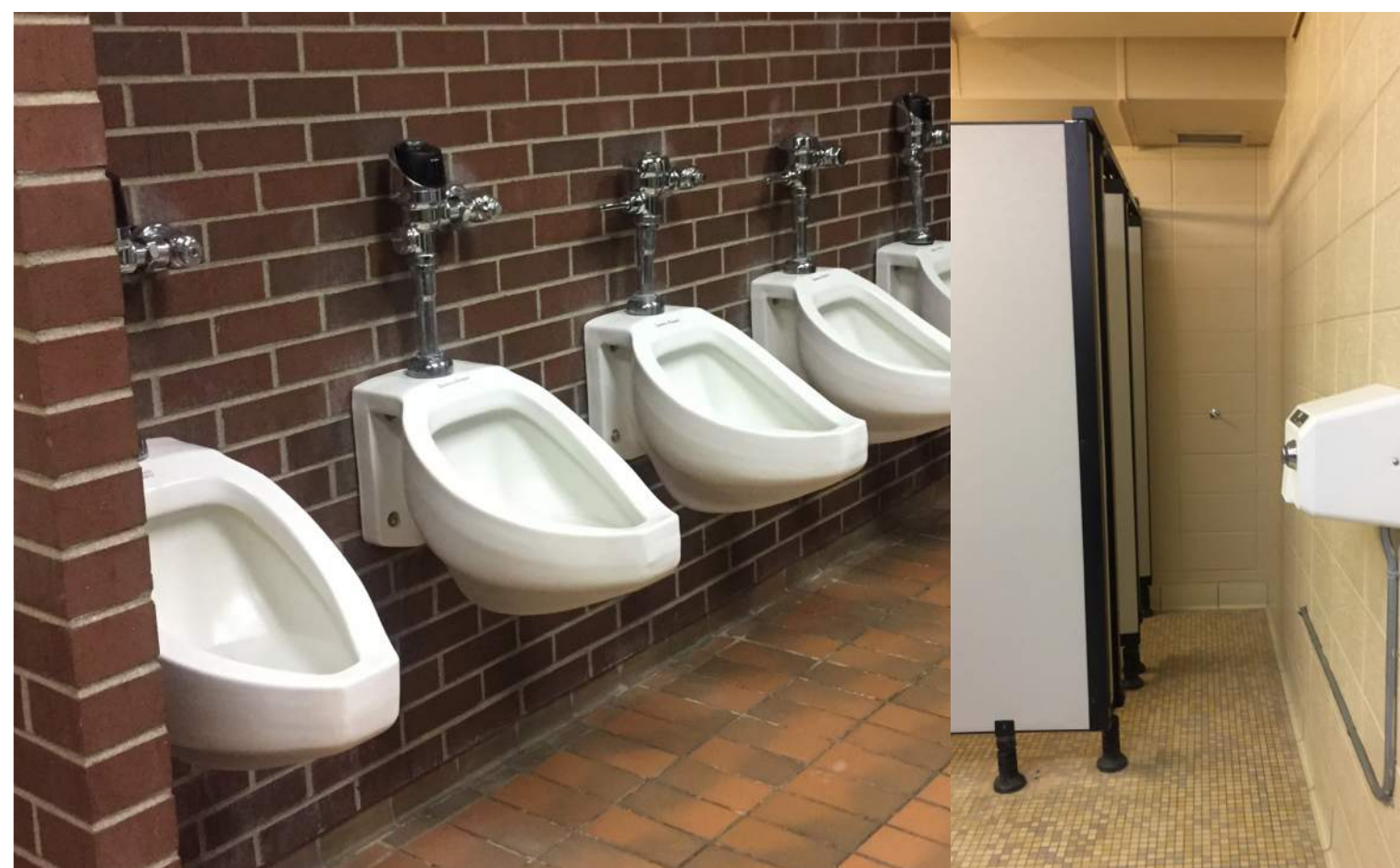
Non-Accessible Bathrooms and Locker Rooms
