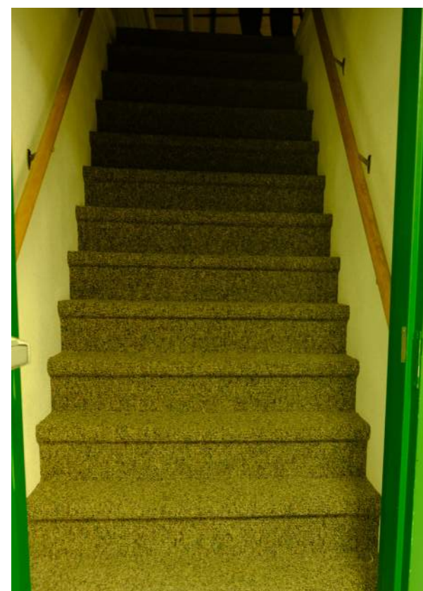
Non-Accessible and Non-Code Compliant Access to Student-Used Spaces
