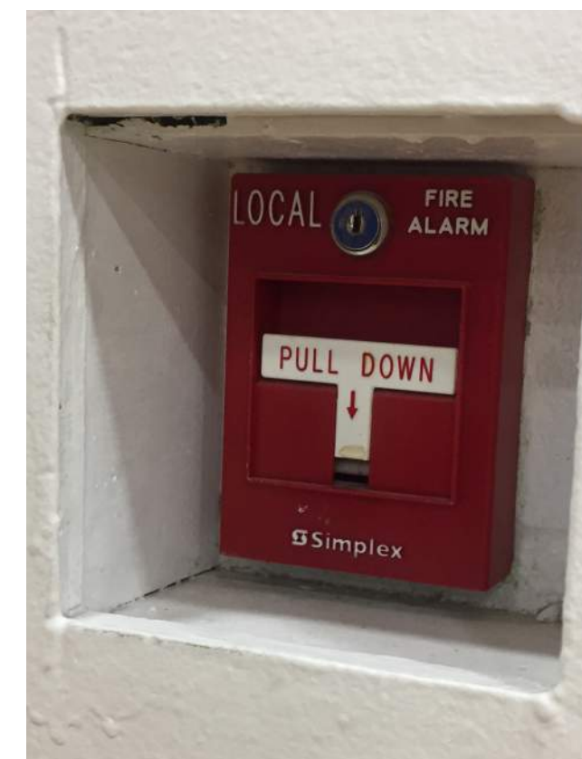
HS Building Without Fire Sprinkler System and Fire Alarm Does Not Meet Code
