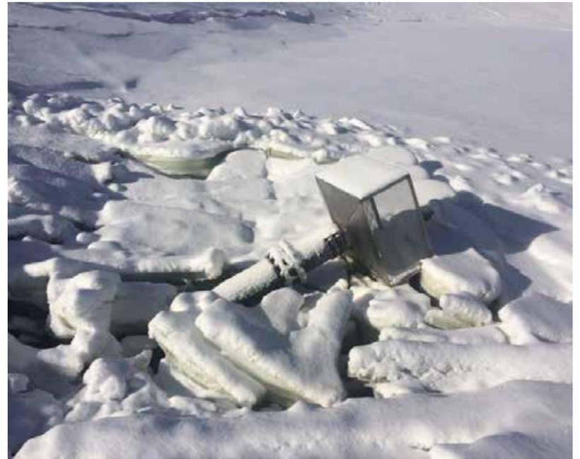
The ice-damaged outlet structure lays at the bottom of the drained pond.
