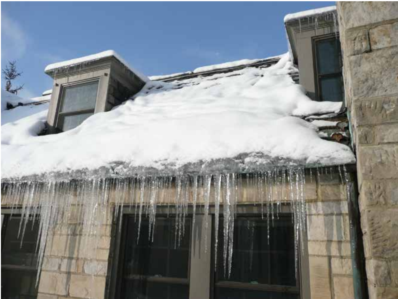
Ice dams often develop this time of year as daily melt-freeze cycles become more common. If left alone, ice dams can allow water to seep into the attic of a home, resulting in wood rot. CC PHOTO
