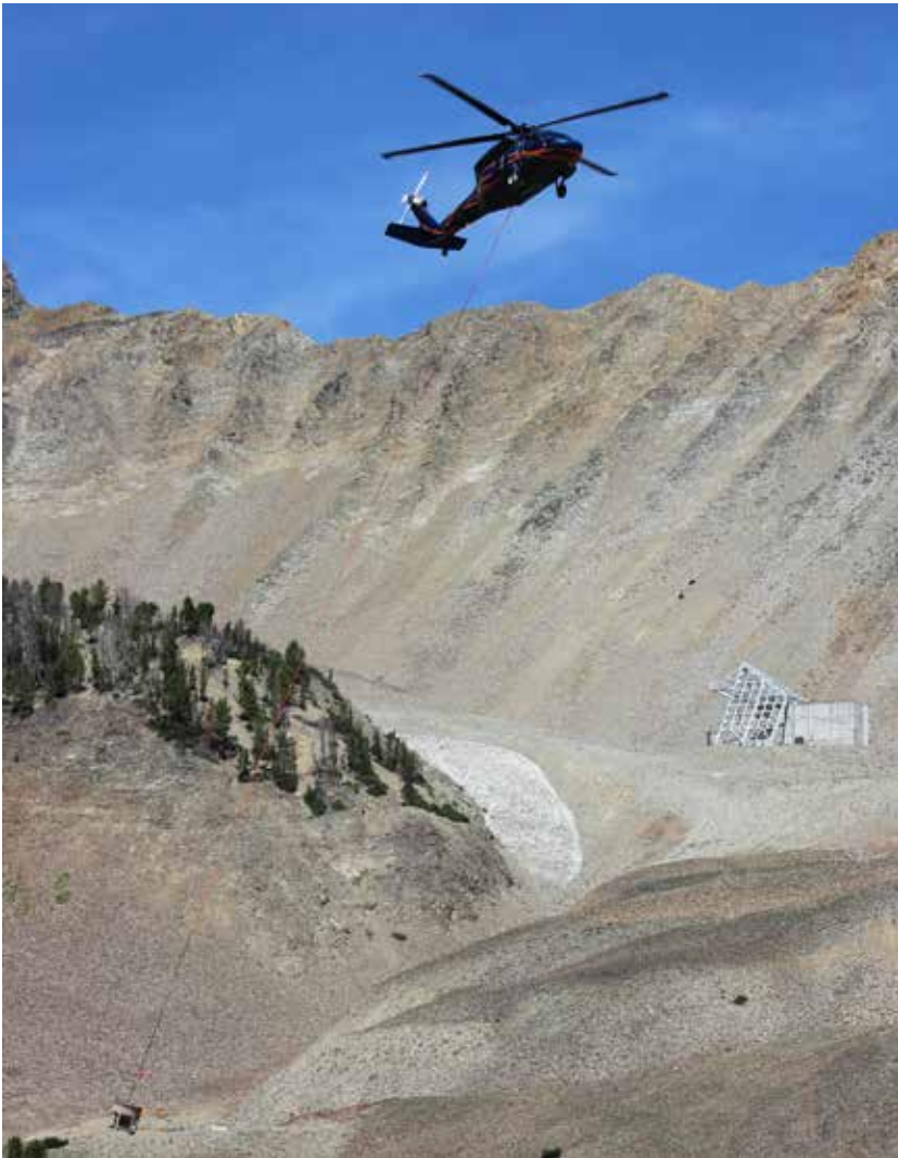
A helicopter flies loads of concrete last summer during the construction of two new chairlifts at Big Sky Resort. The six-place, bubble-enclosed Powder Seeker and conveyor-loading Challenger Triple replaced two aging chairlifts as part of a 10-year, $150 million planned investment by the resort. PHOTO BY TYLER ALLEN
