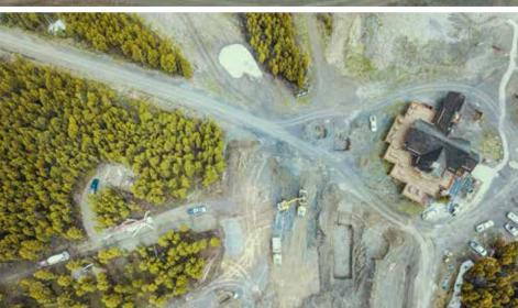
Excavation and concrete work in late June for the terminus of Ramcharger 8 at the top of Andesite Mountain. The first eight-seat, high-speed chairlift installed in North America is planned to open in December, and the heated chairs with blue wind bubbles will be stored underground each night of the ski season to protect their longevity. PHOTOS BY CODY WHITMER
