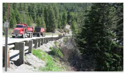
Guardrails effectively keep vehicles on the road and out of the river, but as this segment shows, vehicles striking the guardrails can bend them back as well as loosen the dirt around the posts so that they need to be replaced. PHOTOS COURTESY OF MONTANA DEPARTMENT OF TRANSPORTATION
