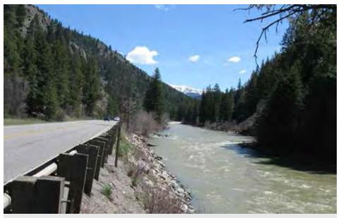
Due to US Highway 191's proximity to the Gallatin River, Montana Department of Transportation had to acquire special permits that mandated replacing the guardrails when the river is flowing at its lowest, beginning in late summer, to minimize impact to the channel.
